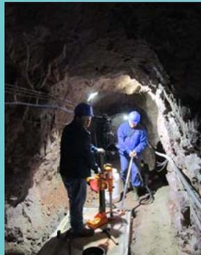
**Figure 3:** Field engineer David Jones and Rudolf Widmer-Schmidrig drilling the second of three holes in the east strainmeter tunnel. The middle cased hole can be seen at the very bottom.
